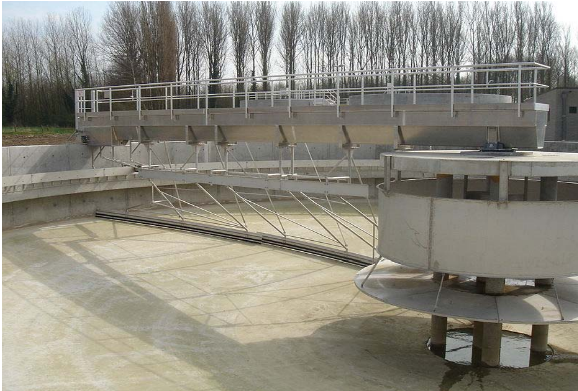
An empty sedimentation tank at the treatment plant in Merchtem, Belgium
