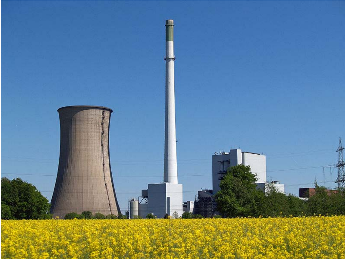
Cooling tower at Gustav Knepper Power Station, Dortmund, Germany
