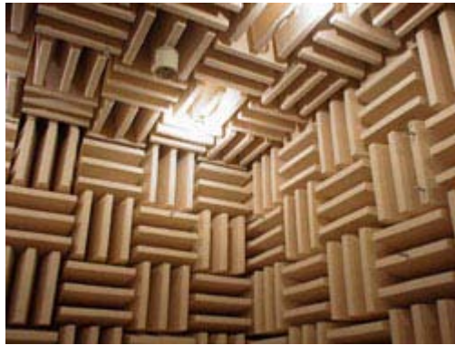
A anechoic chamber, showing acoustic damping tiles used for noise absorption
