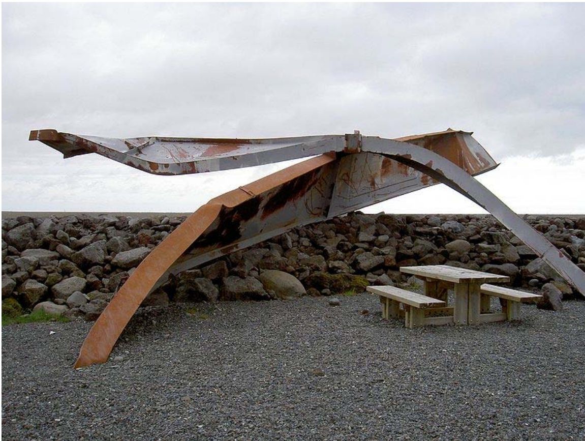
Remains of a steel bridge in Skaftafell National Park after a glacial outburst
