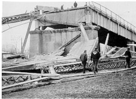
The collapsed Silver Bridge, as seen from the Ohio side
