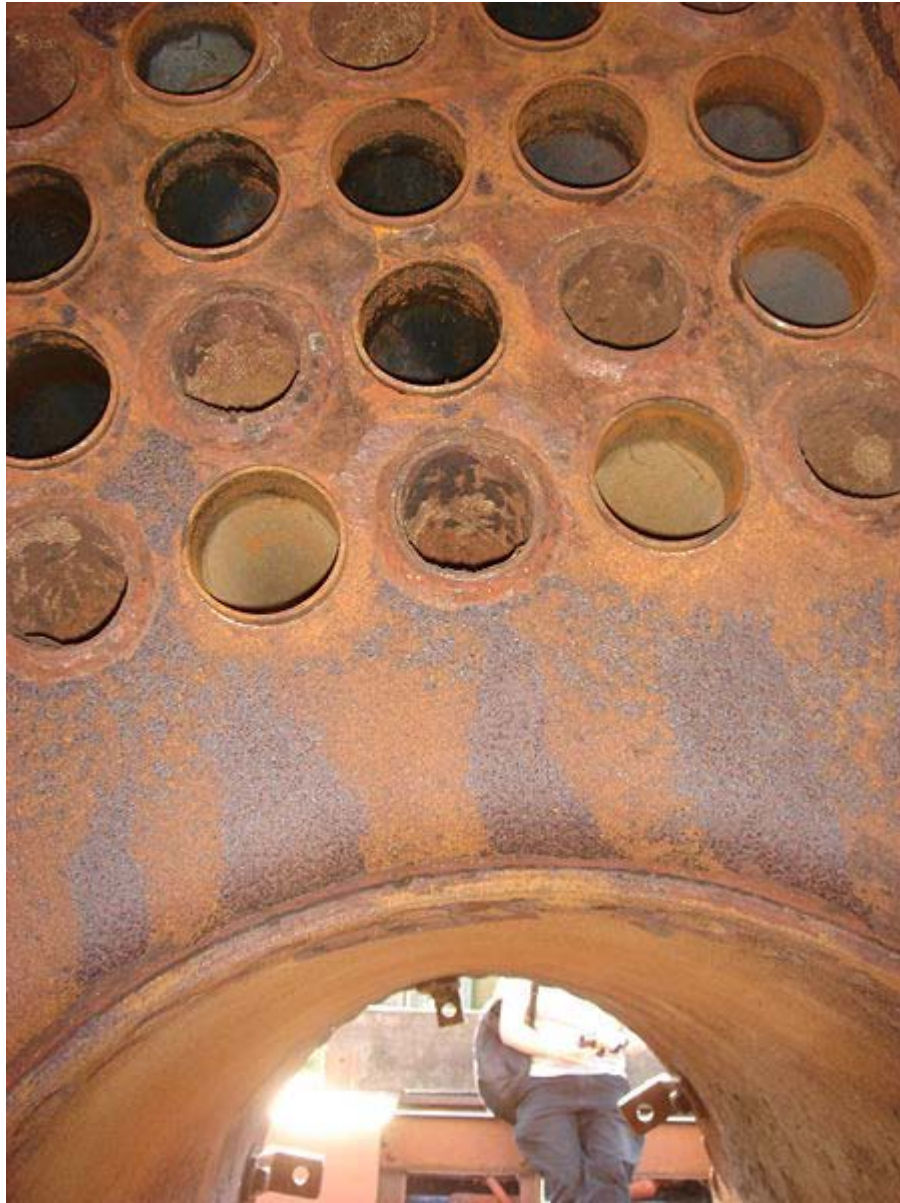
Inside the combustion chamber, looking up at the tubeplate
