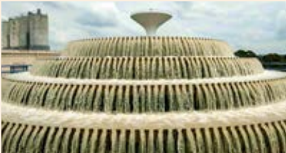
Treatment Plant Optimise treatment process by removing or reducing contamination per water quality target
