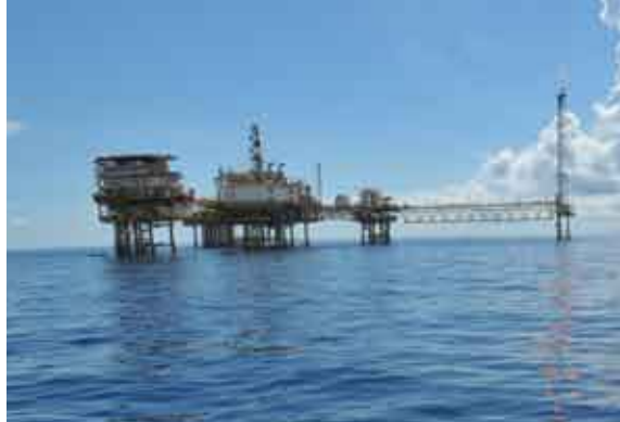
The Erb West platform located offshore Sabah
